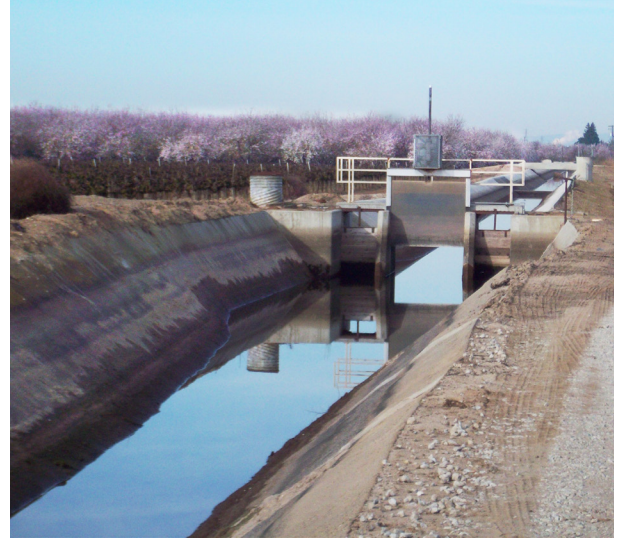
The district's main canal feeds 28 laterals, which account for hundreds of miles of ditches, pipes and gates throughout the county. Blossoming in the background are acres of almond trees, one of the region's primary crops.
