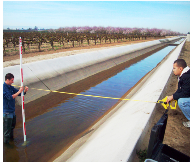
SonTek Product Manager Mike Cook and HydroScientific West representative Diego Davis prepare a SonTek-IQ installation site in one of the SSJID laterals. User friendly mounting brackets allow them to install the SonTek-IQ by simply inserting two bolts 12.7 cm (5 in) apart along the center line of the channel. The orientation of the slots on the mounting plate to allows users to orient the instrument in the direction of flow. Ultra-low power consumption allows for smaller solar panels and batteries – making monitoring less conspicuous.
