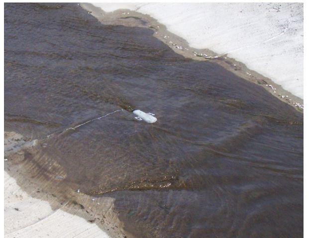
The SonTek-IQ can accurately measure flow in as little as 3 inches of water is extremely valuable to SSJID when measuring smaller canals or drains.
